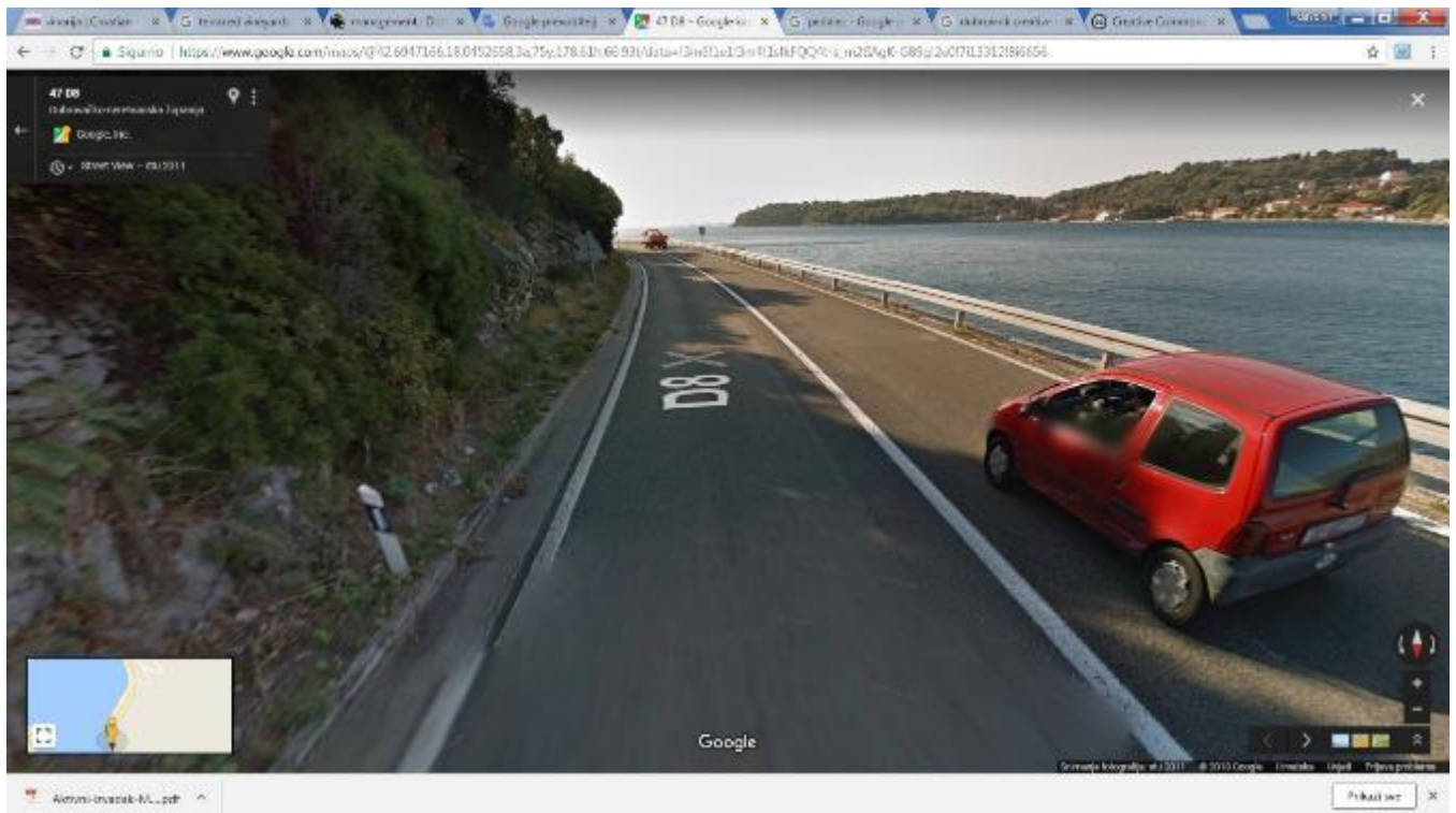
Section from Zaton to Dubrovnik bridge with high traffic
