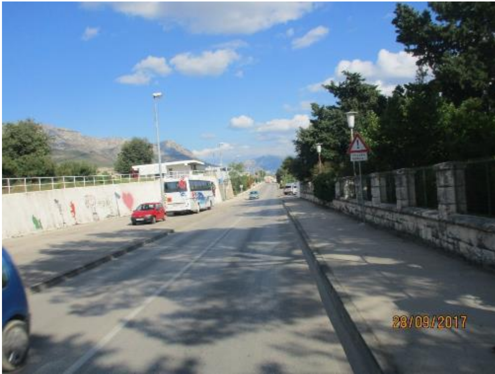
Kaštel Gomilica: road with high traffic and two wide sidewalks
