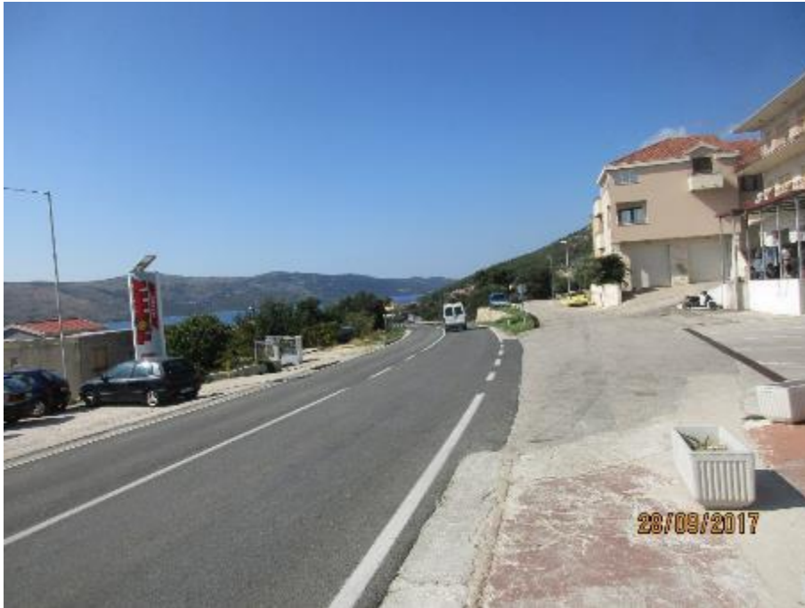
Very dangerous crossing road D8 close to Seget Vranjica
