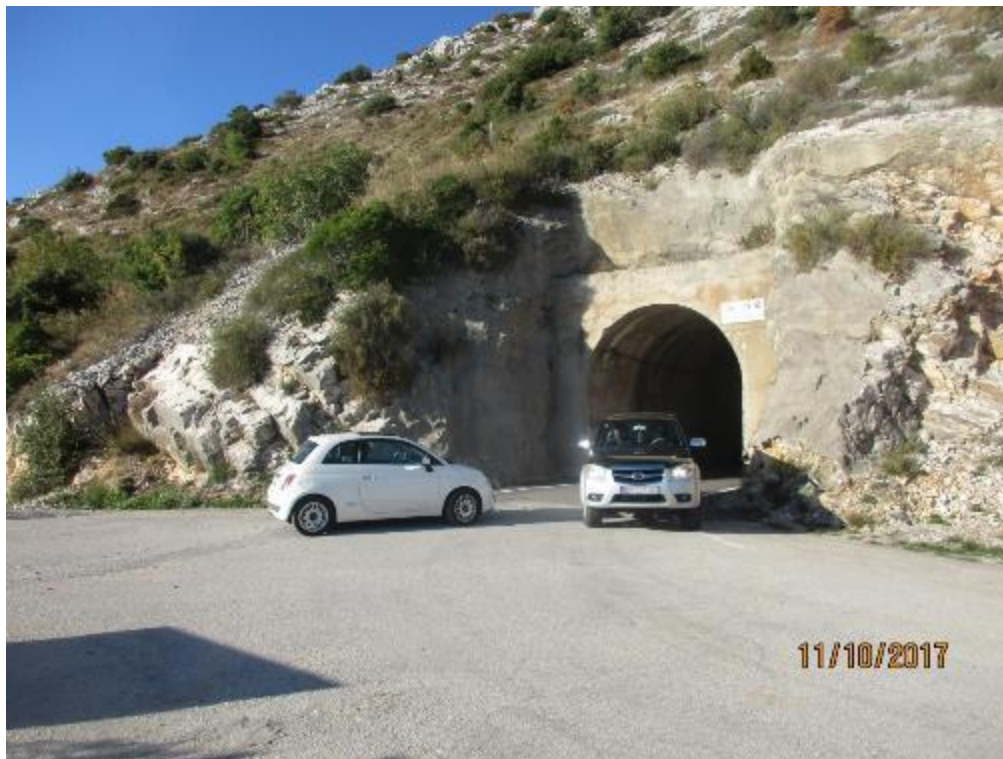
Dingač tunnel, length 400 m, still some cars, but weak light in the tunnel
