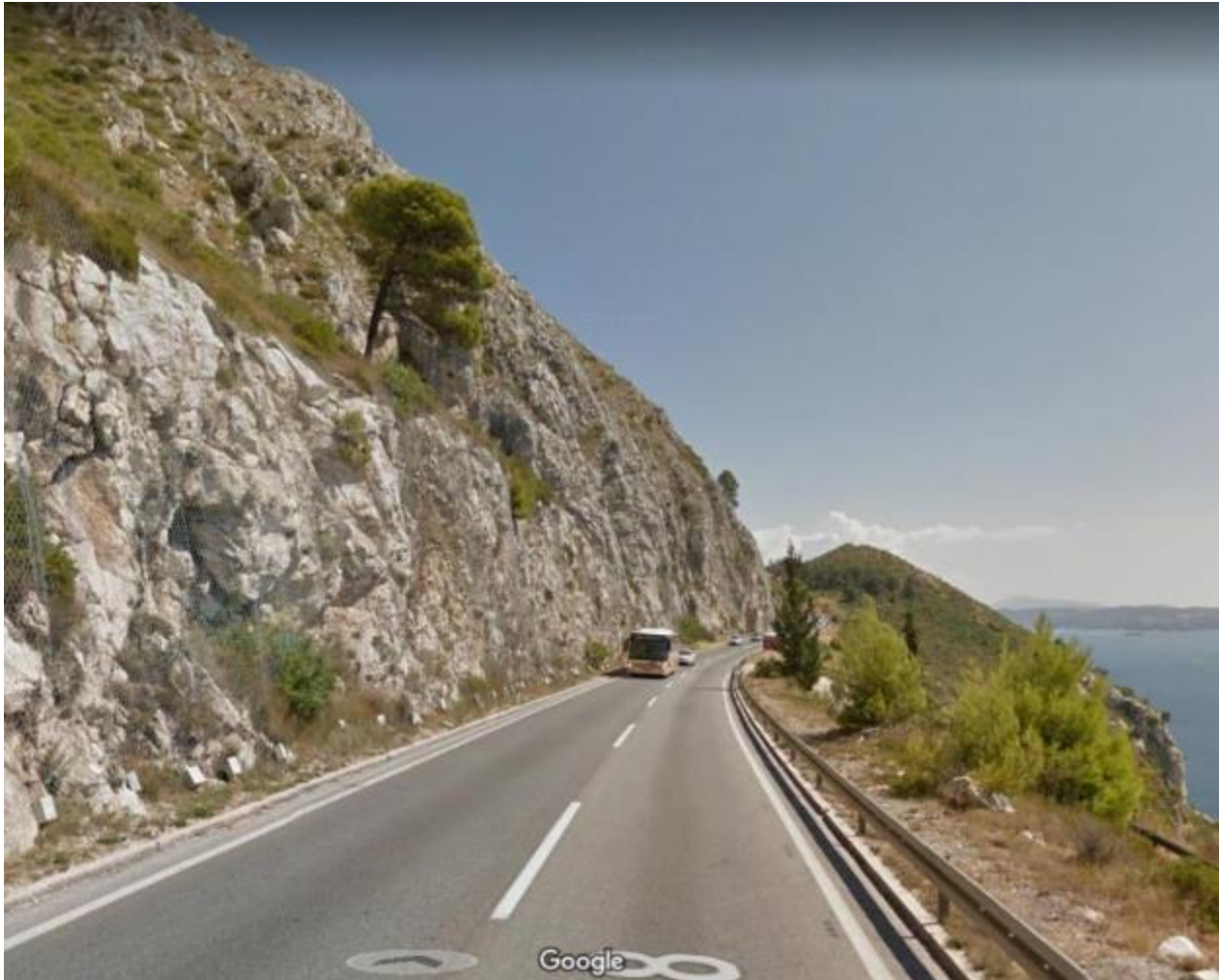
Road with very high traffic close to Dubac (table row 31) Extension of the road by the bicycle path on such section is extremely expensive
